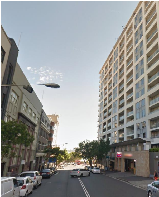
PICTURE 5 – 50 MURRAY STREET LOOKING NORTH
