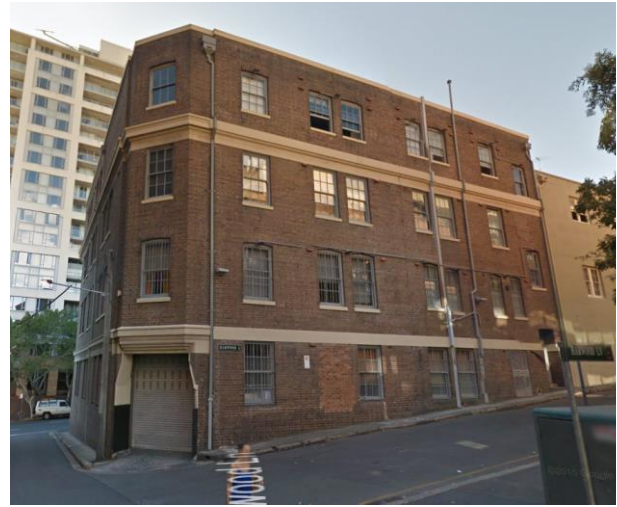
PICTURE 4 – 47 MURRAY STREET LOOKING EAST
